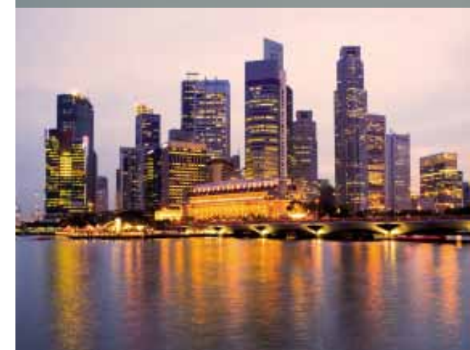
Singapore. Building homes, hotels and offices
